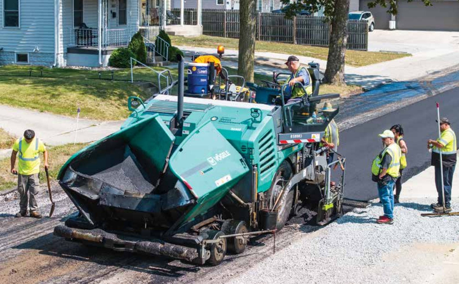
The milling crew paves a road with a VÖGELE SUPER 1703-3i wheeled paver.
