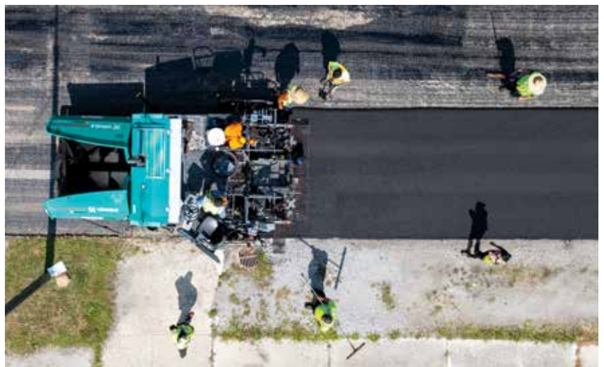
The VÖGELE SUPER 1703-3i wheeled paver is in the 8-foot class.
