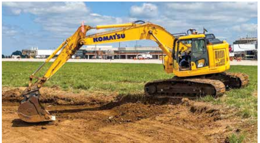
An operator uses a Komatsu PC238USLC tight tail swing excavator equipped with Smart Construction 3D Machine Guidance to cut out a retention pond.
