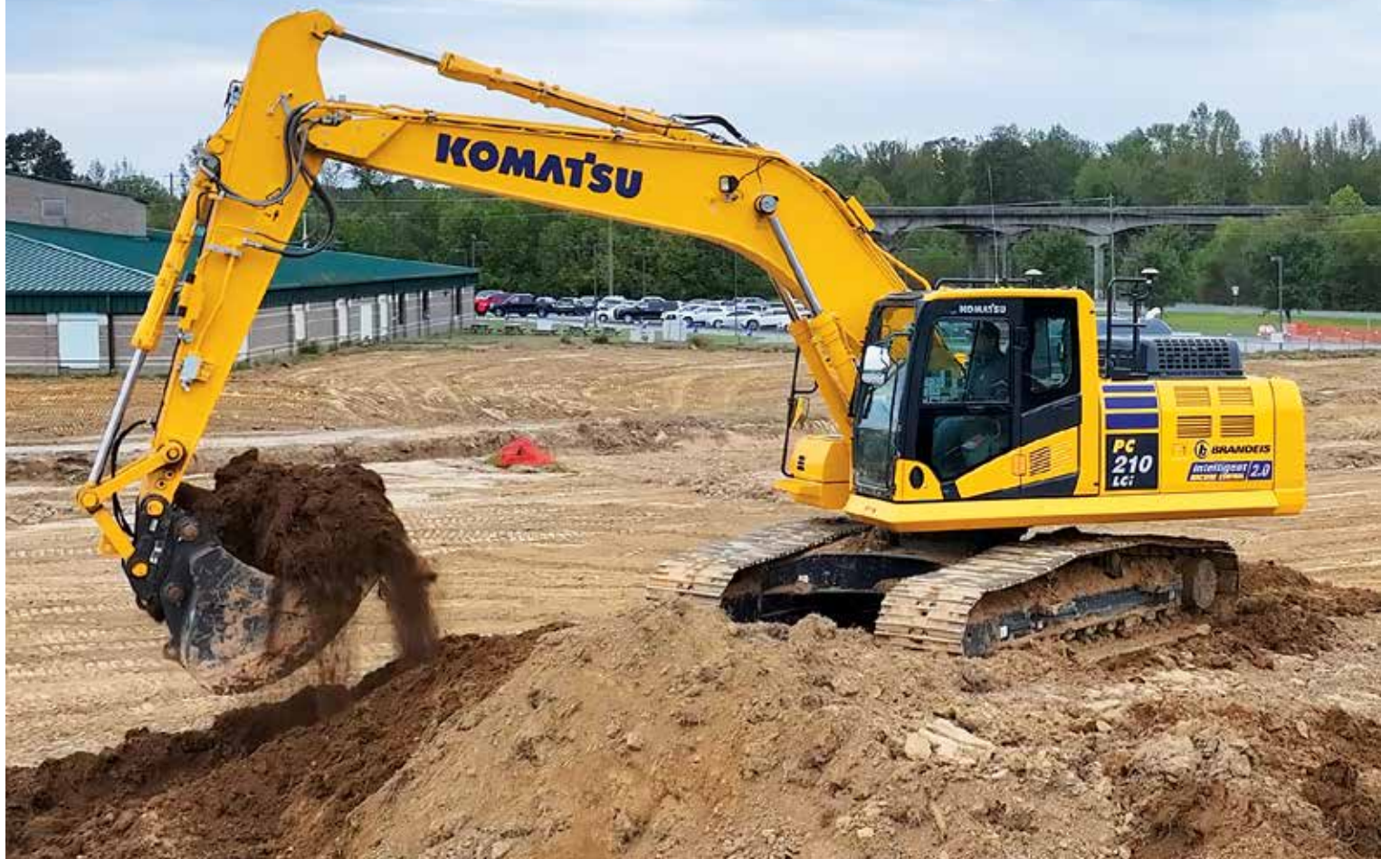
An operator picks up a bucket of material with a Komatsu PC210LCi-11 IMC excavator.
