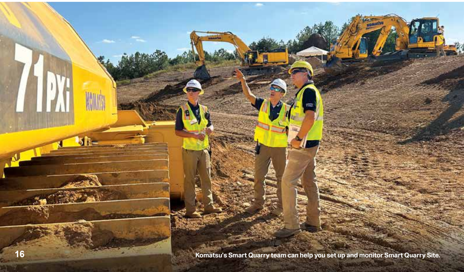
Brandeis Machinery's Curtis Slack (left) and Dean Excavating's Hunter Dean run the excavators.
