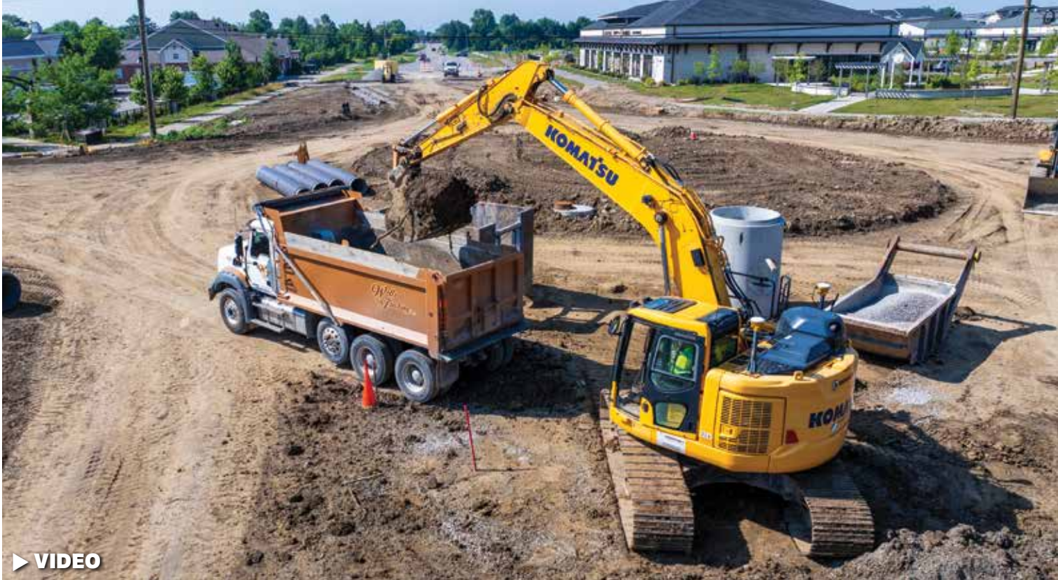
An operator loads material into a truck with a Komatsu PC238USLC tight tail swing excavator.
