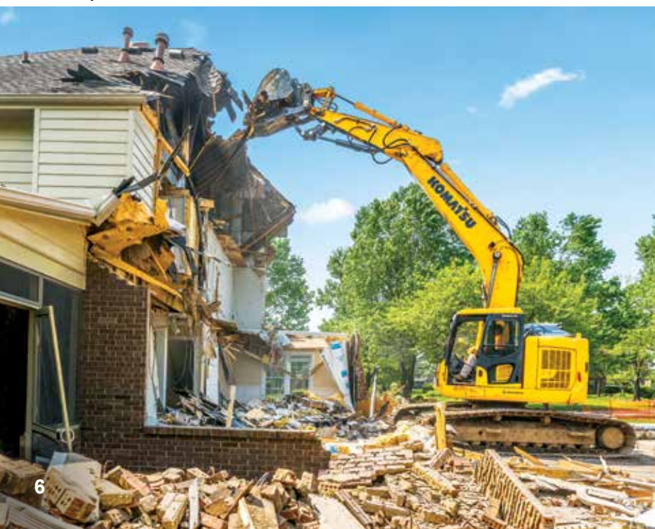
An operator tears down a roof with a Komatsu PC238USLC-11 excavator.
